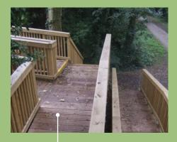
**RESIN AGGREGATE INSERTS** All the deck boards on the ramps and the steps had double centralised anti slip aggregate inserts incorporated to aid with grip.
