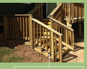
**TIMBER SPECIFICATION** North European Redwood was used throughout the project treated to Deckbuilders standard specification of Tanalith E to Hazard Class 4
